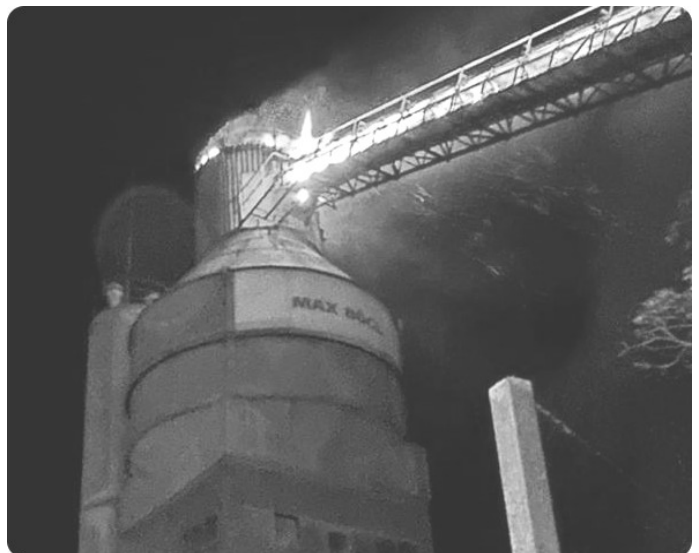
02.09.24: repression fails to stop the attacks in Munich – huge Max Bögl concrete plant hit, 7 pieces of heavy machinery torched, conveyor belt ignited & starts to burn the mixing silo, millions of euros in damages (among other projects, Max Bögl worked on the Grünheide factory; see Cars as Cameras)
