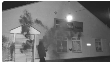
12.01.25, Glasgow, UK: windows smashed at hi-tech Parker-Hannifin production facility, paint sprayed inside
