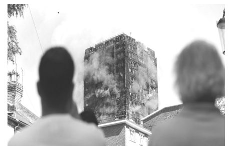
14.06.17, London, U.K.: Grenfell flats, after repeated legal threats to the residents who warned likelihood of fire
