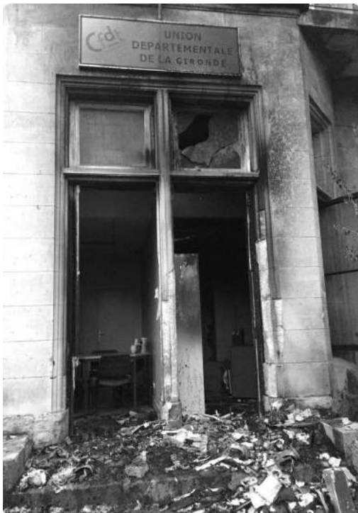
Bordeaux, France: CFTD office heavily fire-damaged a week after the events in Paris
